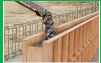
Concrete forming and base for laminating.
